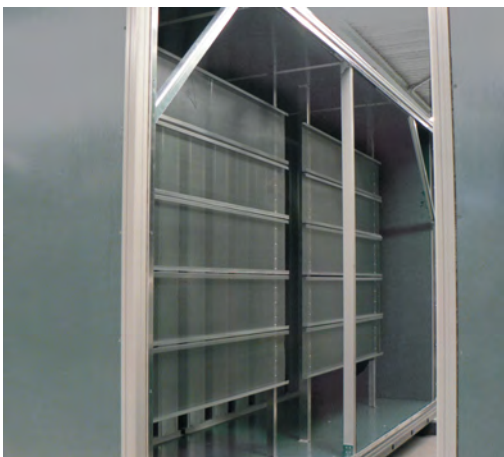
Air Distribution Screen
